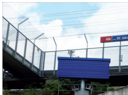
Stadionbahnhof St. Jakob, Basel (BS) Vandalenschutznetze / Filets anti-vandalisme / Vandalism protection nets
